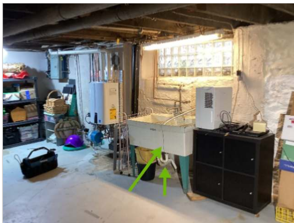
Tub loose and flex line on trap
