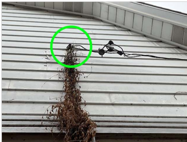
Loose weather head with overgrowth
